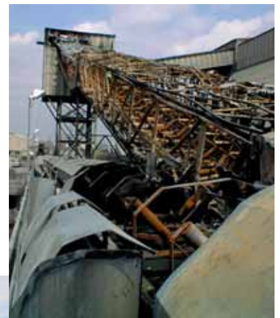
Main picture: a Dunlop BV XS conveyor on the left stopped the spread of fire while, inset above, belts with inadequate fire resistance can be expensive!
