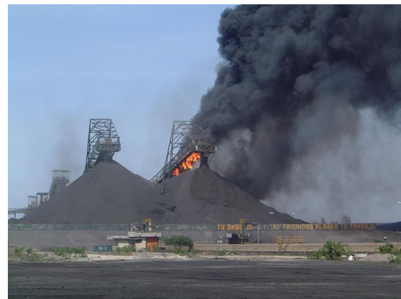
No conveyor belt is fire proof
